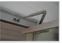
Hydraulic door closer which can hold the door 90° in position
